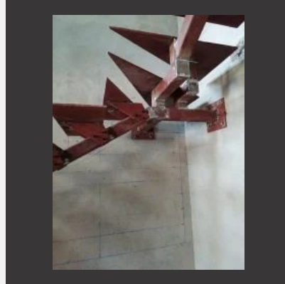
Sheet Metal Works
