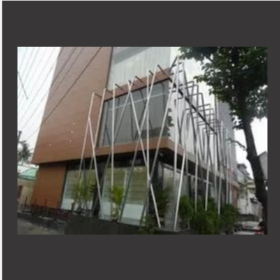
Structural Glazing Spider Fittings
